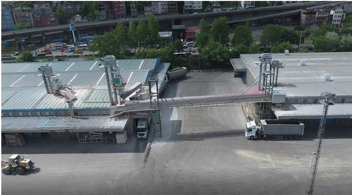
GENERAL VIEW OF THE PROCESSING SYSTEM
